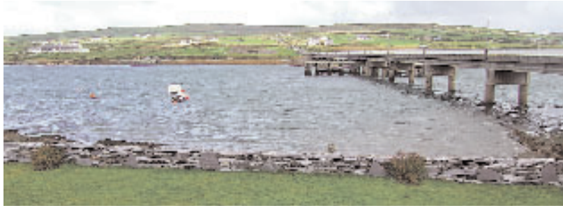
FIG 16. Bridge from Portmagee to Valentia, County Kerry. (Geograph: Jonathan Billinger)
