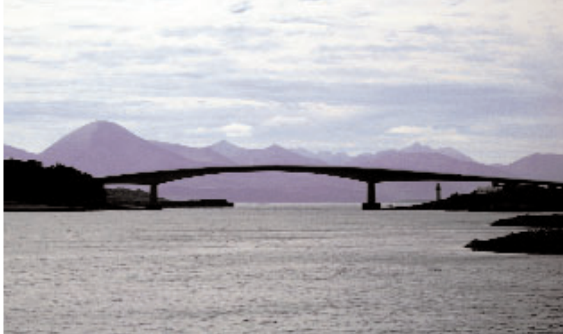
FIG 13. The Skye Bridge, connecting Skye to the mainland across Loch Alsh. (Martyn Gorman)
